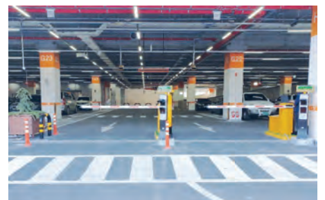
▶ Pyeongtaek Samsung Parking Tower
